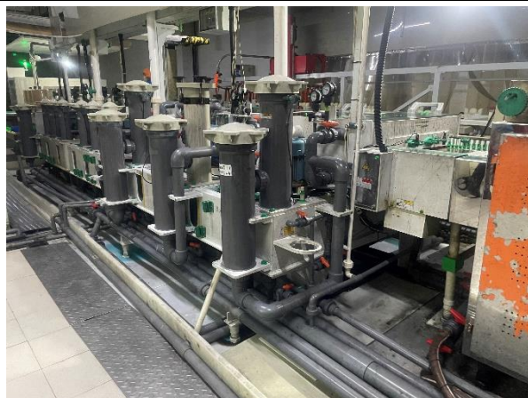
1层镀铜车间管线设置于托盘上
